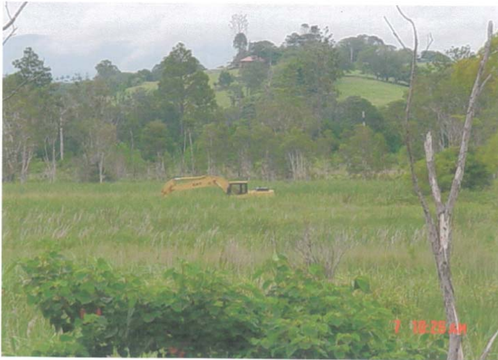
Completed drainage works in North South SEPP 14 - Coastal Wetlands. Upstream.
