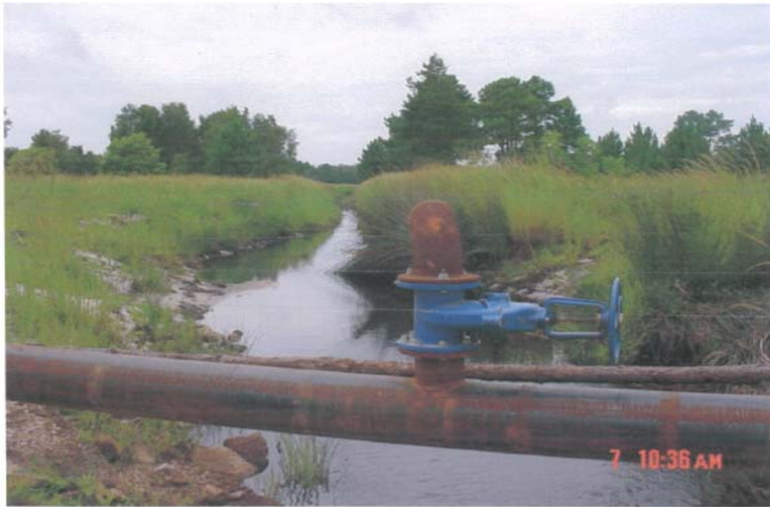
Drains created from North South SEPP 14 - Coastal Wetland.
