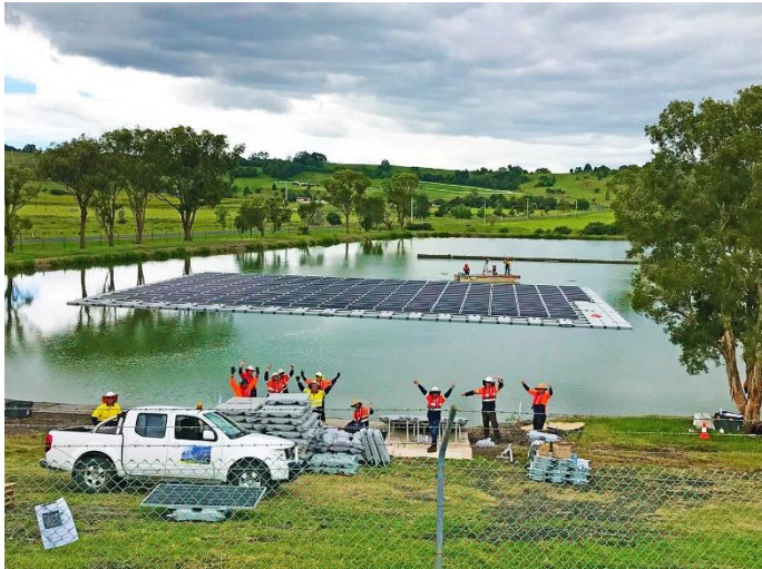
FIGURE 5: LISMORE CITY COUNCIL'S FLOATING 100 kW SOLAR
