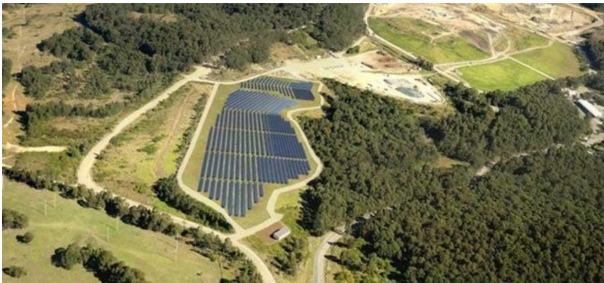
FIGURE 3: THE CITY OF NEWCASTLE'S 5 MW SOLAR FARM 1
