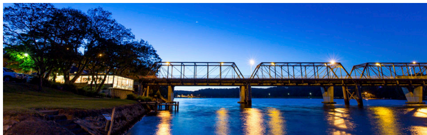
Nowra Bridge, Shoalhaven.
